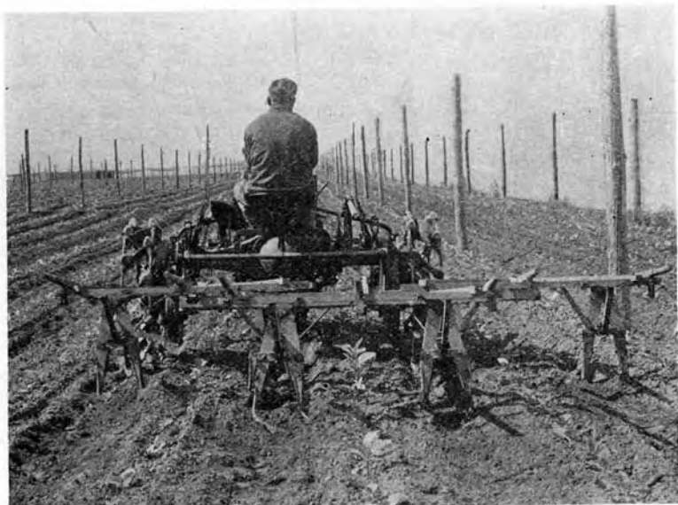
FIGURE 24. Prout hoes drawn by tractor. Rear view.
