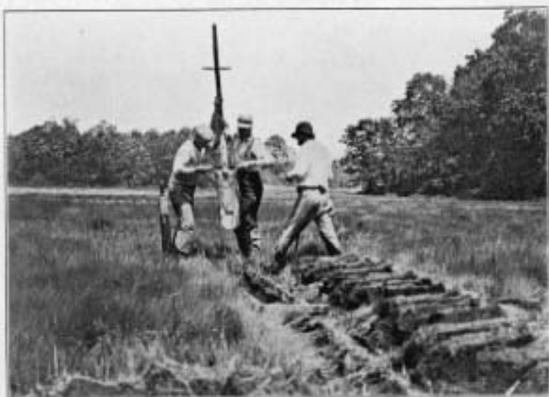
a. Draining the salt marsh. The spade raised ready to be plunged into the peat.
